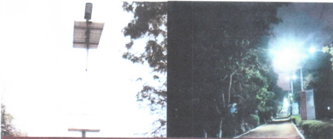
Solar Street Light Installation at the Campus
