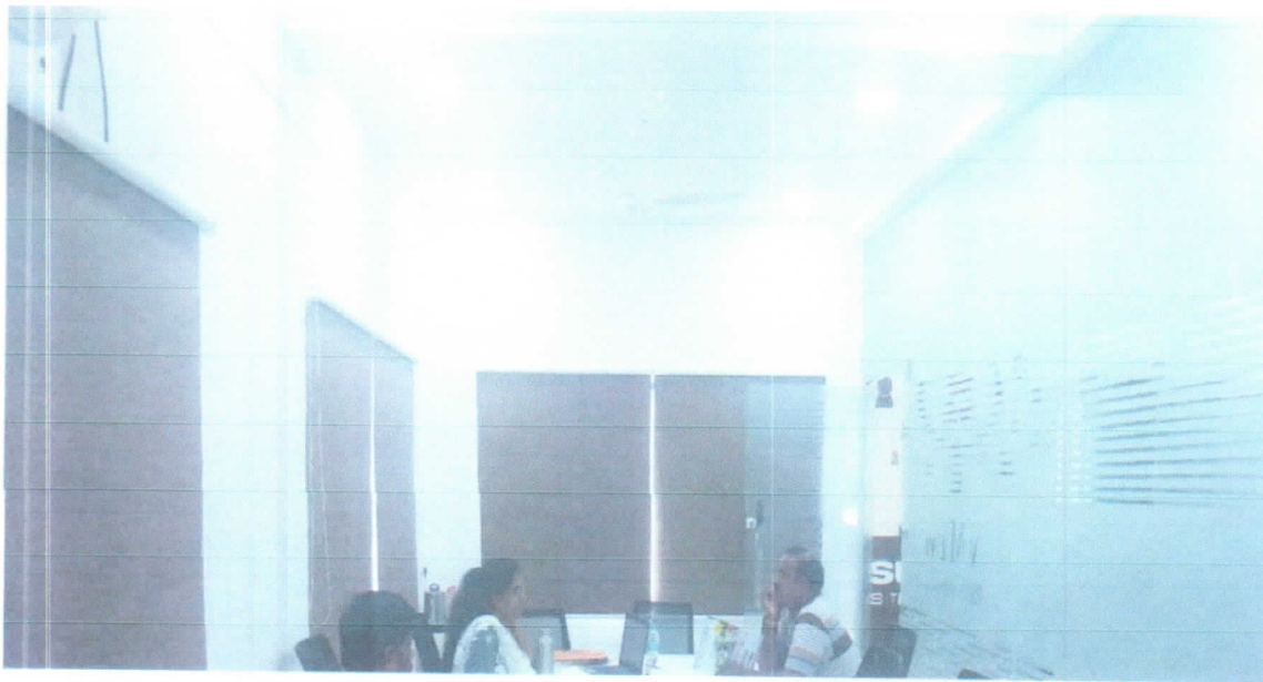
Use of LEDs in Placement office Board Room
