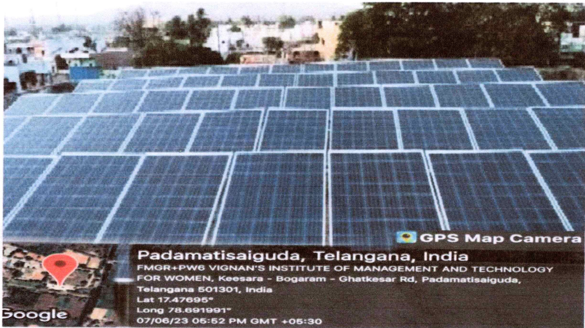
Solar Power Panel on the rooftop with a capacity of 50kW
